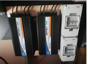
keep things working comfortably on hot days. They come in 30 and 60 Amp versions and where higher amps are required, several can be used in parallel when hooked up to independent panel sets.
