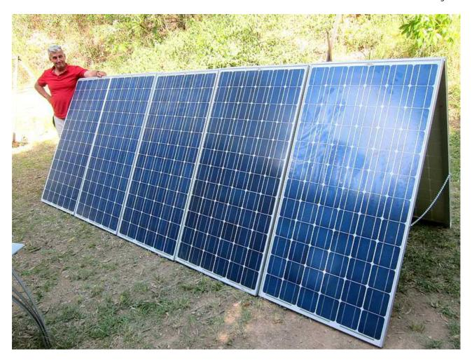
A-Frames made up of 185-195W panels generally put out around 300W per cloudy day. This makes calculating the amount of A-Frames required, an easy task.
