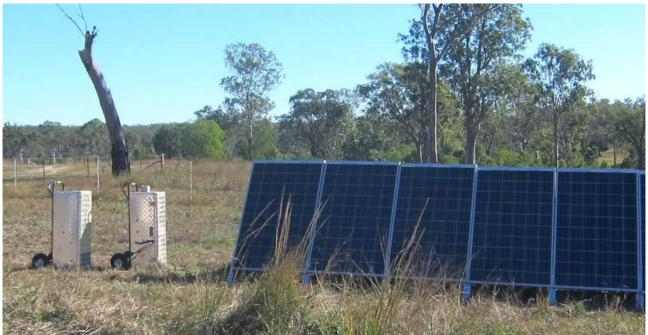
The boxes,.. which have the batteries, solar charger, inverter, fuses etc., built in and wired up, are wheeled into position and simply clicked onto the solar array extension and switched on. It's that easy. The boxes can either be used in an upright space saving position in garages or small rooms, or laid down and pushed under floors, shelves, into the back of larger campers or under the solar A-Frames.
